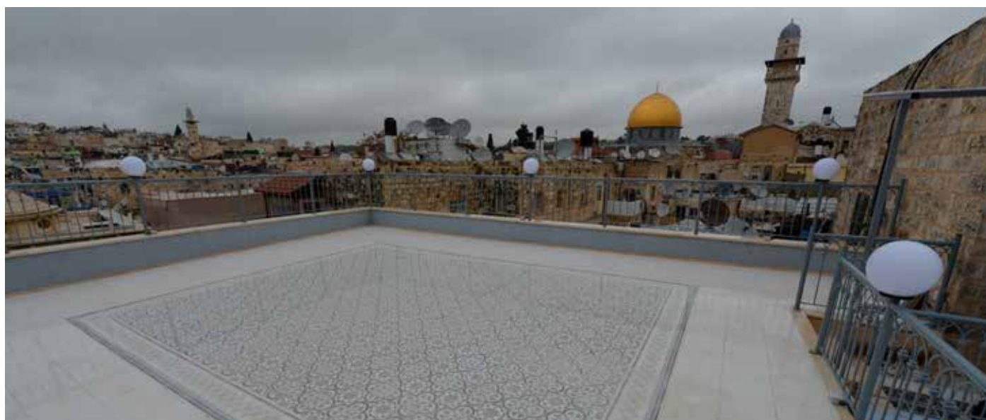
Khalidiya Library Annex Renovation in Jerusalem - Old Cities of Jerusalem Revitalization Program (OCJRP)
