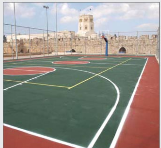
20- Burj Al Laqlaq playgrounds after rehabilitation
