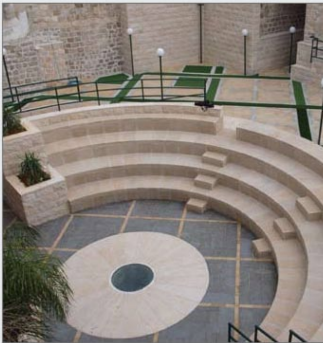
21- Habaleh Square after rehabilitation
