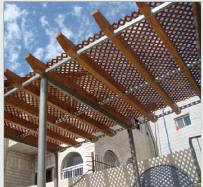
19- Al Ansari library after restoration
