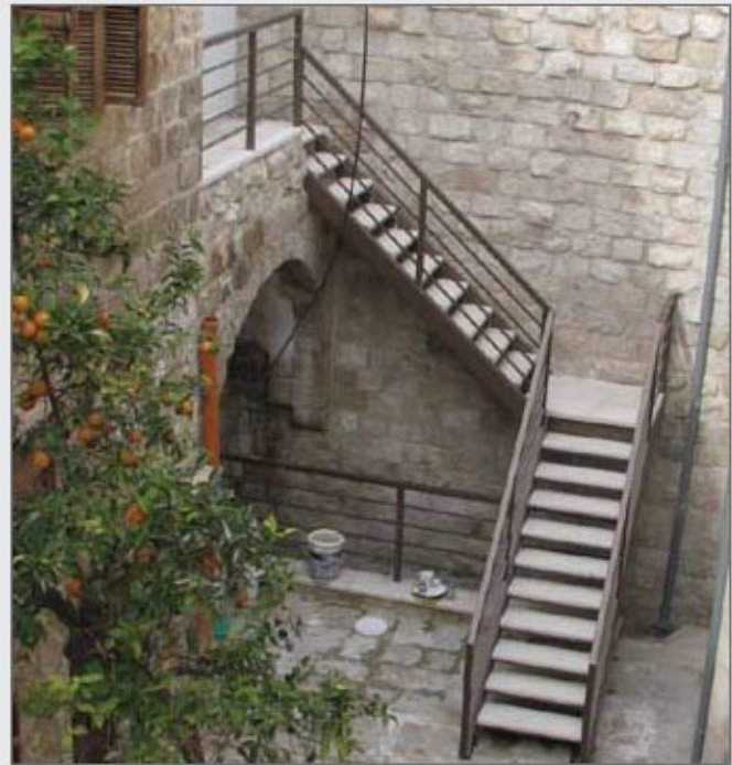
21- Hesh Al Shobi complex after restoration
