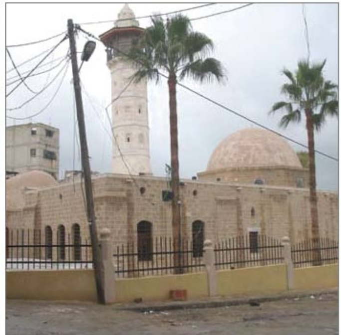
15- General view of Al-Sayyed Hashim Mosque - Gaza
